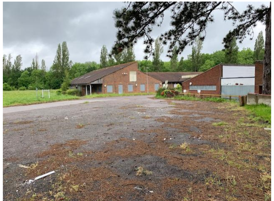
C. View east from the car park to derelict buildings
