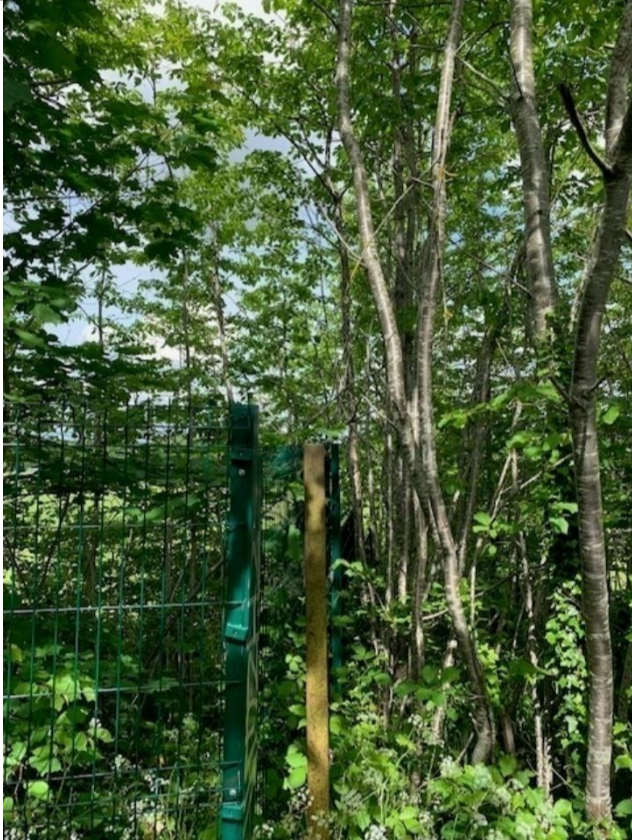
F. Boundary fencing between the site and adjacent field to the west of the site.
