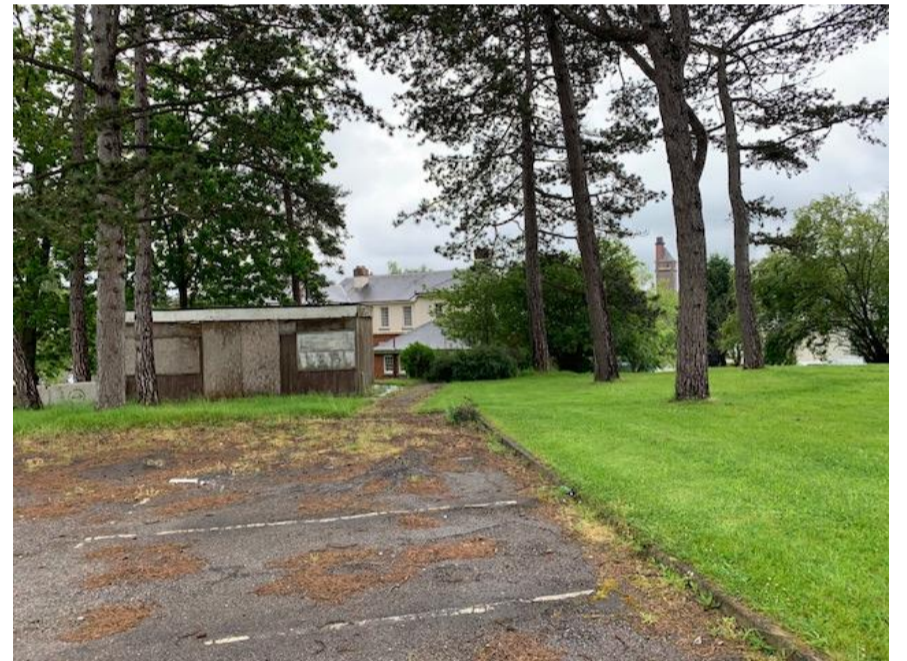
A. View looking south onto the site from the north. Derelict shed on the edge of the site, next to now unused car park
