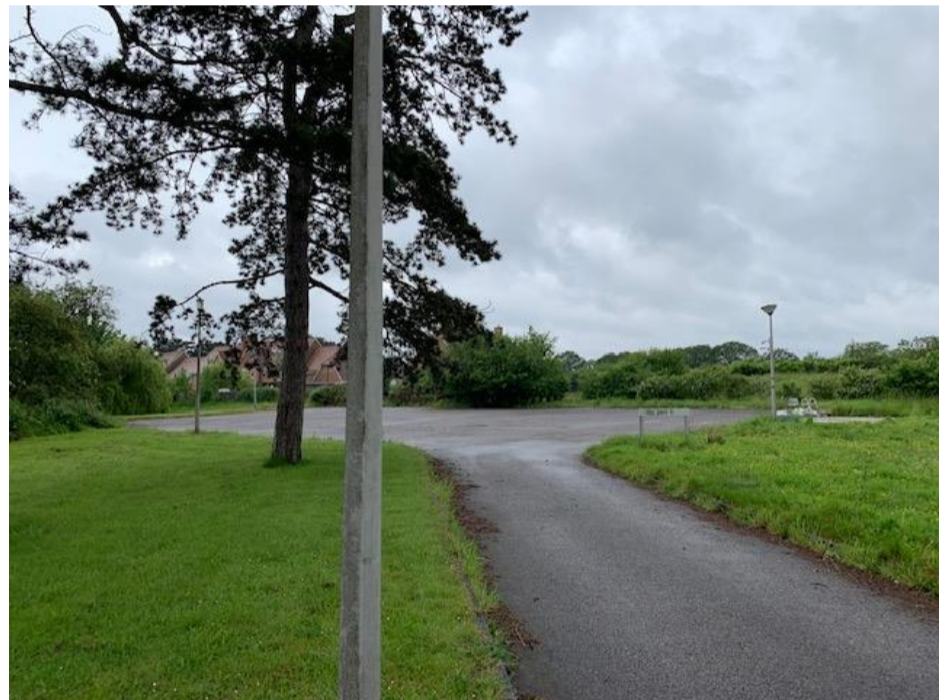
A. Derelict car park to the west of the site
