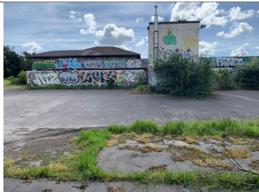
G. View of derelict buildings from footpath along the northern boundary (FP104)
