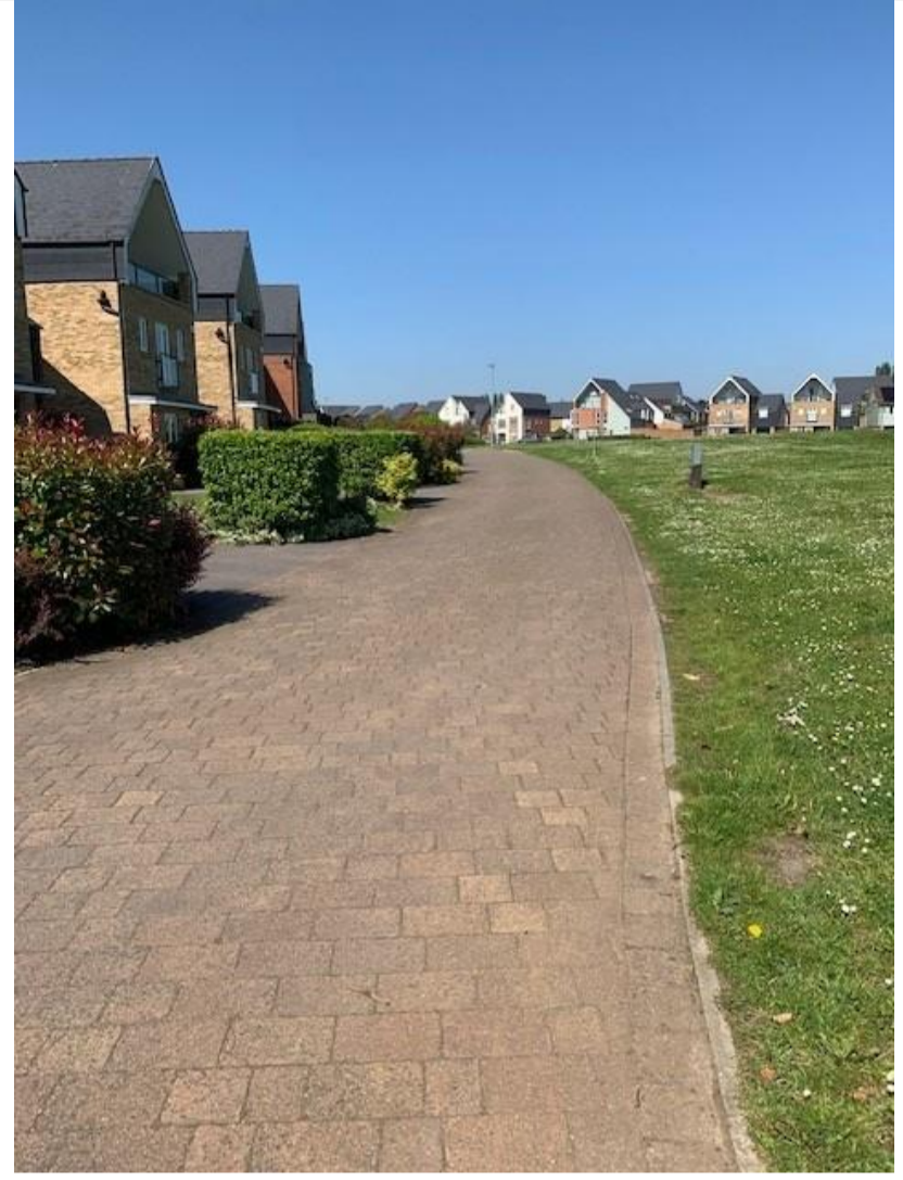
B. View of St Ebba's estate from Maple Close, looking NW
