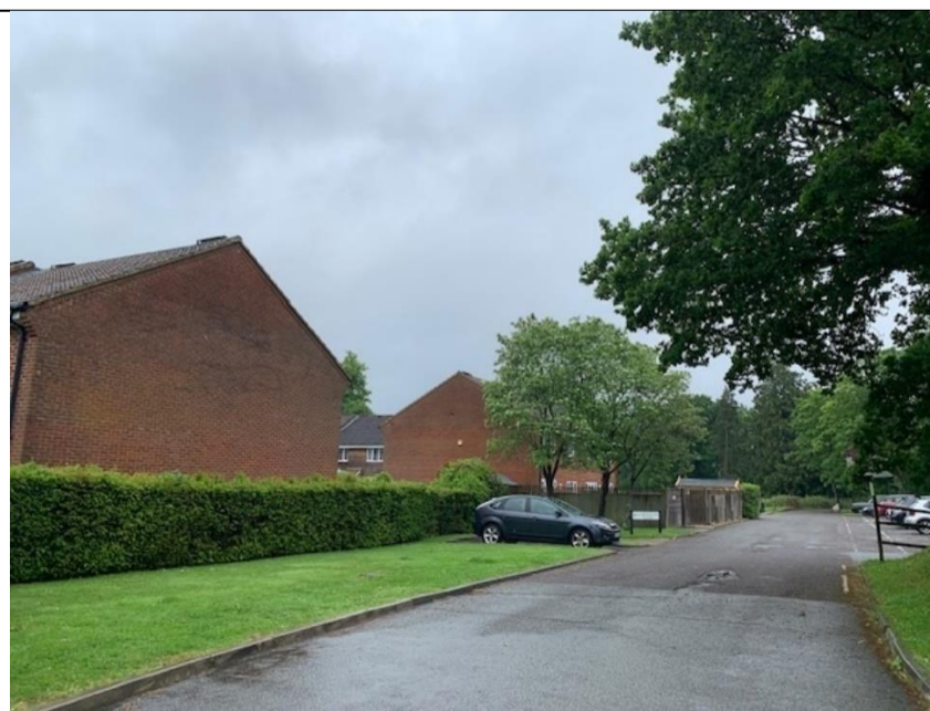
C. Cuddington Glade residential estate to the north of the site
