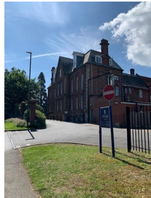
D. Back entrance from College Road
