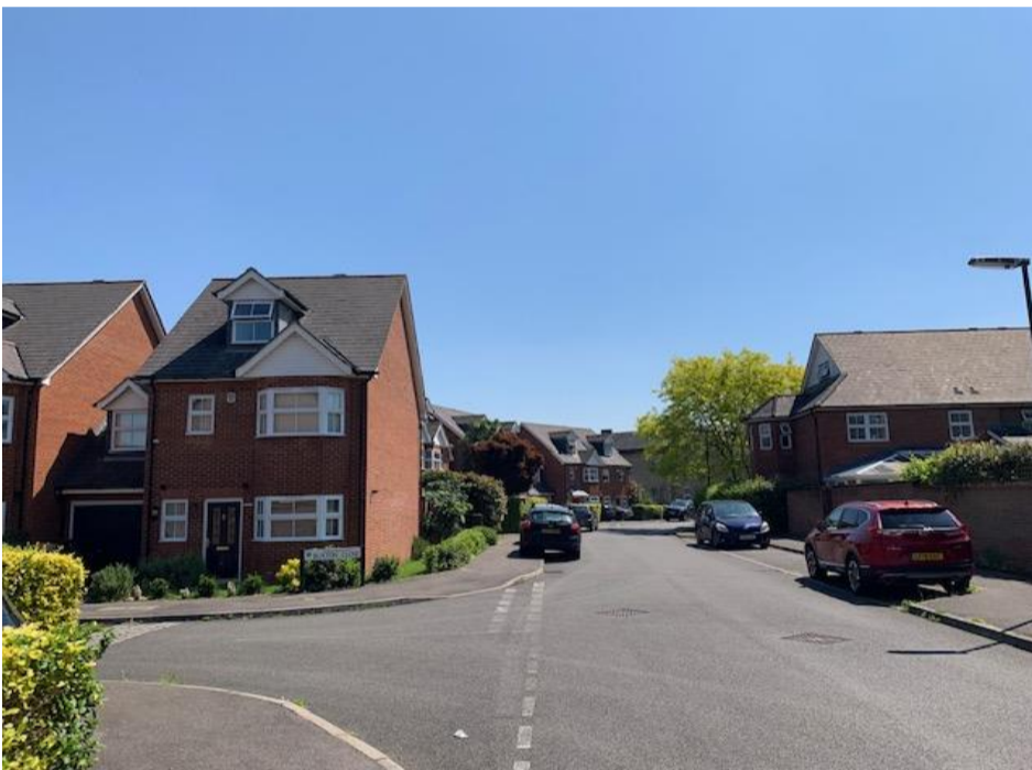
C. Detached and Semi detached properties along Horton Crescent (West)
