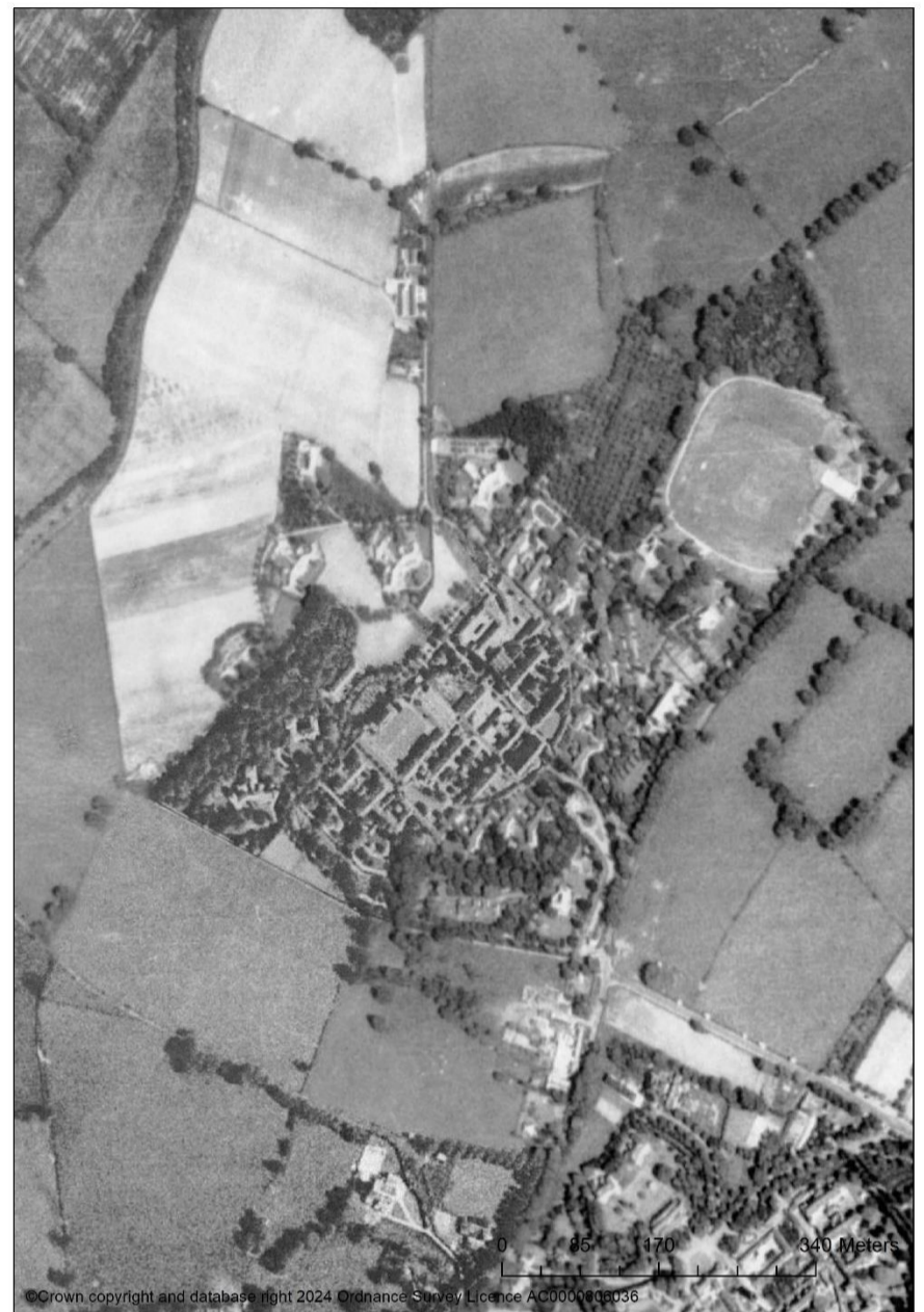
Historic aerial photo of the former Long Grove hospital
