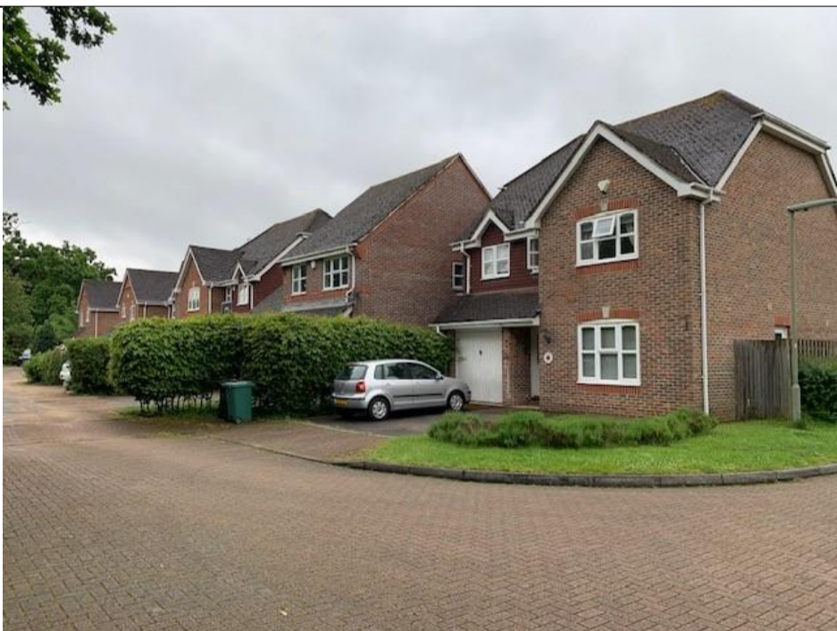
E. Residential found units located in the eastern parcel
