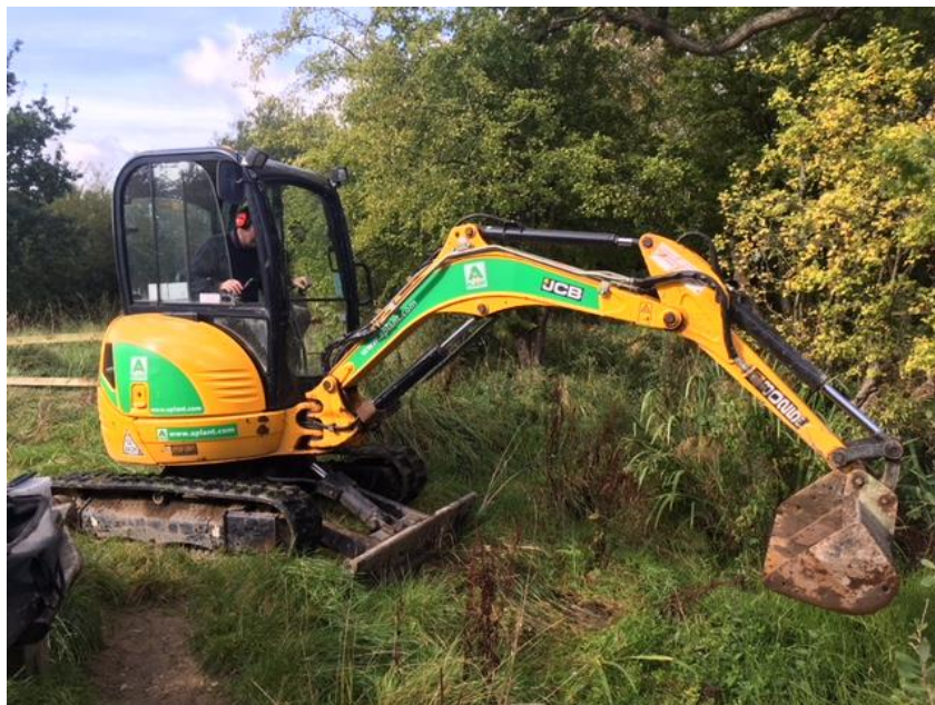
Lower Mole Partnership about to begin work to desilt Field Pond in Horton Country Park LNR September 2017
