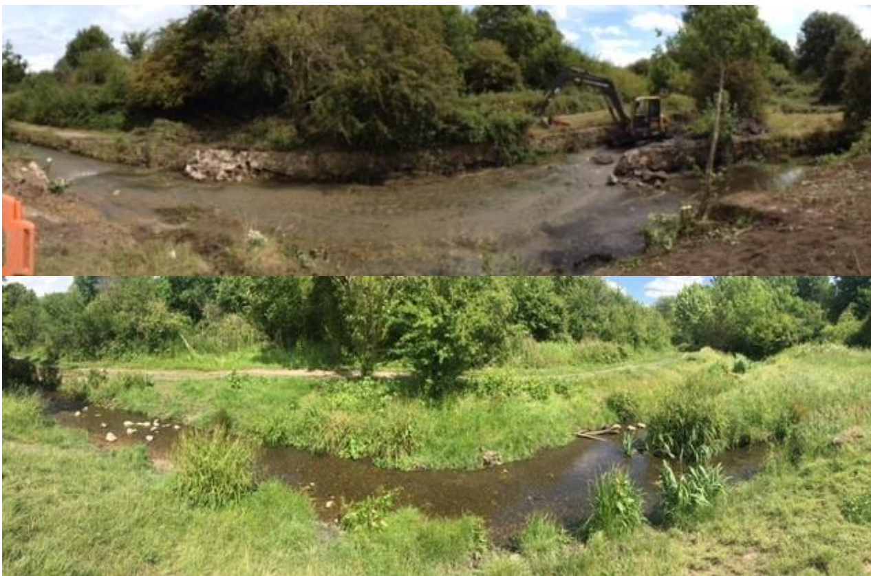
Hogsmill LNR, confluence of the Hogsmill River and Green lanes Stream shown in August 2014 with work commencing to remove walled banks and concrete bed and the naturalised banks and bed in June 2017
