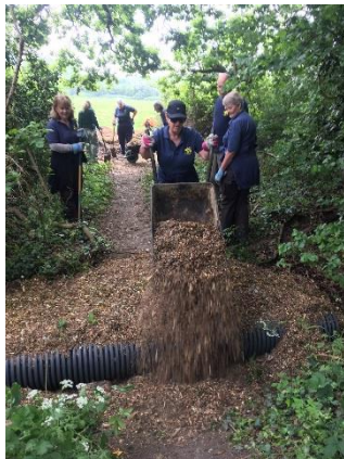
EEBC Countryside Team Volunteers constructing a wood chip path in Horton Country Park LNR spring 2017
