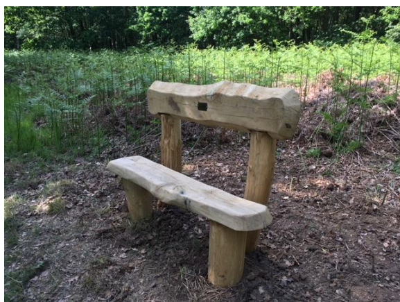
The completed bench!
