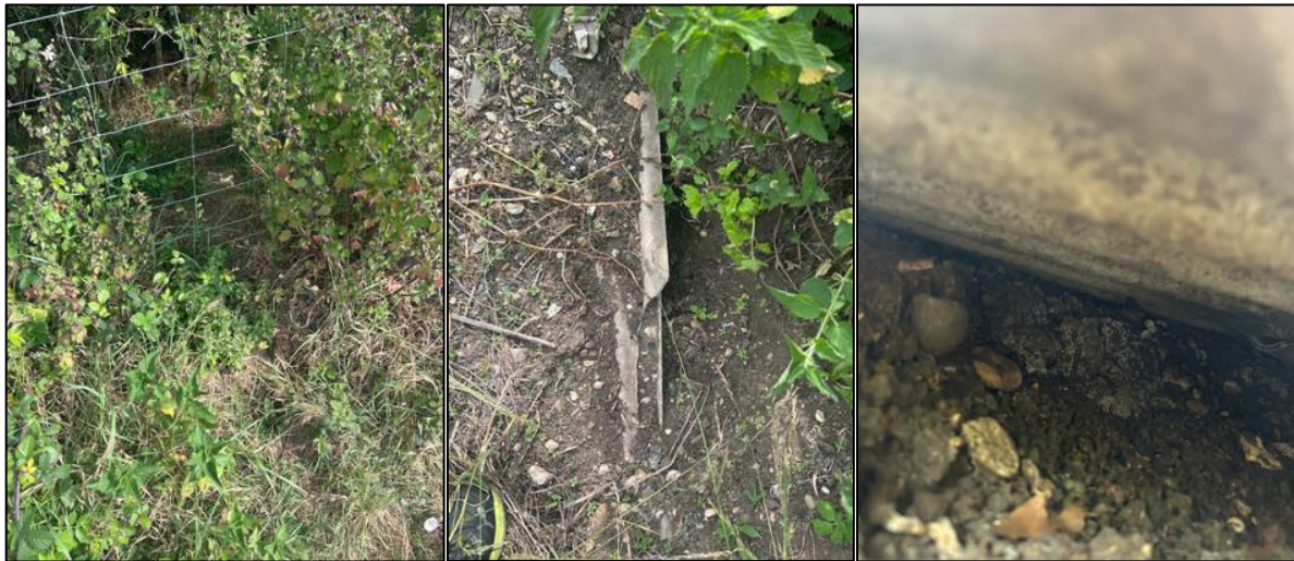
Photographs 6-8. A badger push through under a stock fence, with a guard hair found at TQ2065457800 and an excavation under a chrysotile sheet that that does not extend beyond around 40cm at TQ2067657805.
