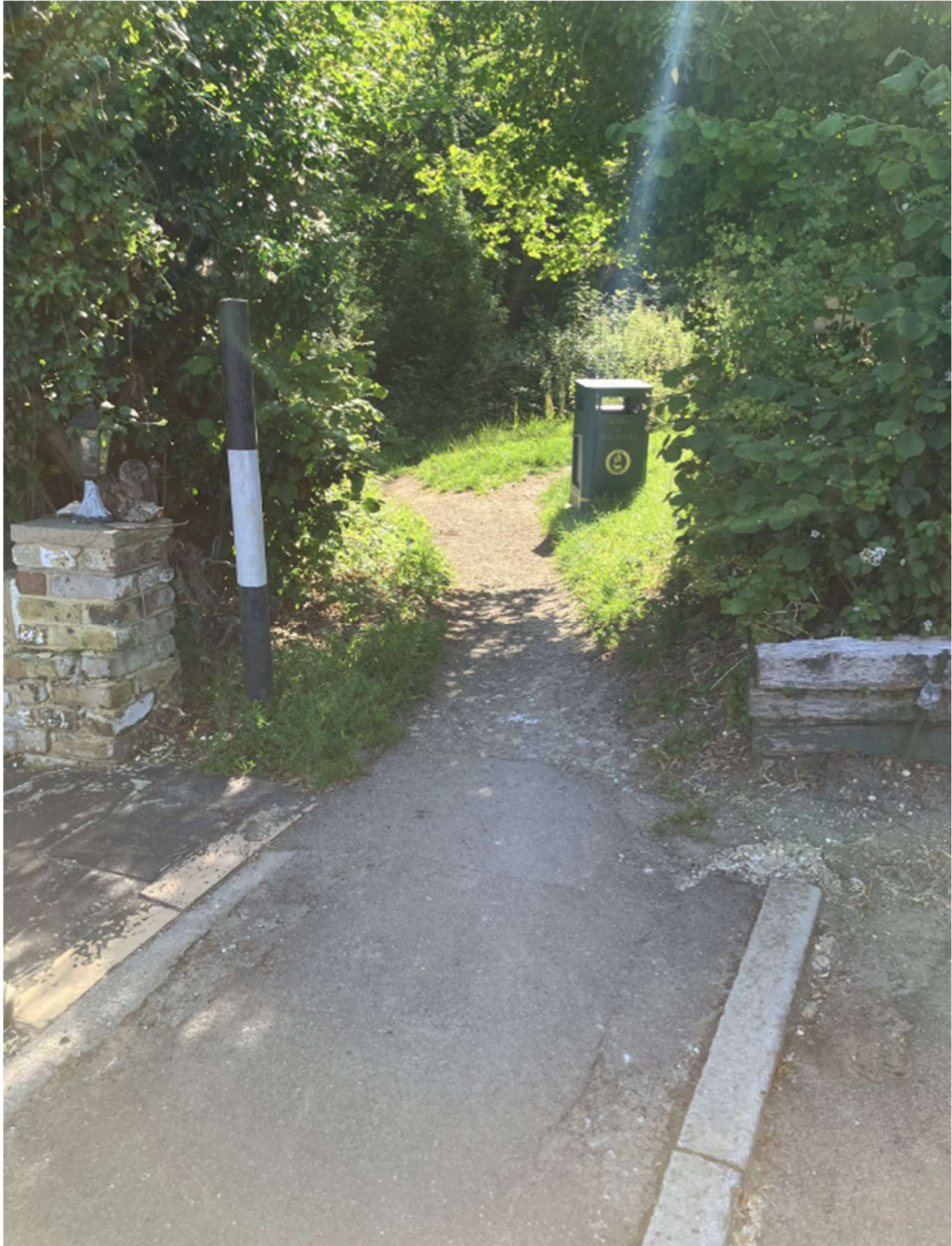
Photograph 2 - Footway link at Beaconsfield Road - 19 th June 2026
