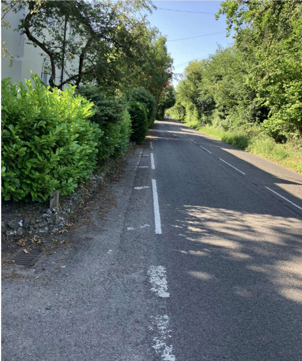
Photograph 10 -View south- Headley Road/Chalk Pit Road junction – 19 th June 2026
