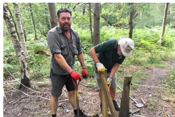
Volunteers from the Lower Mole repairing a squeeze gate on Epsom Common LNR July 2018
