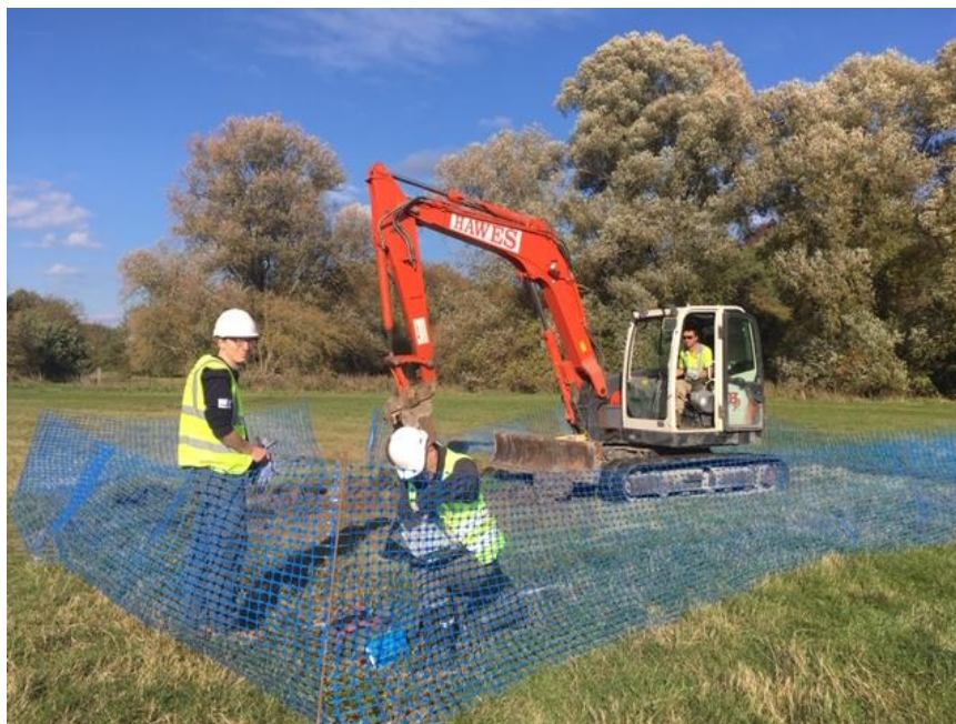
Hogsmill LNR, South East Rivers Trust staff digging test holes on Chamber Mead October 2018
