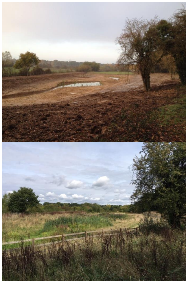
New balancing pond in Horton Country Park LNR just after construction January 2016 and September 2018
