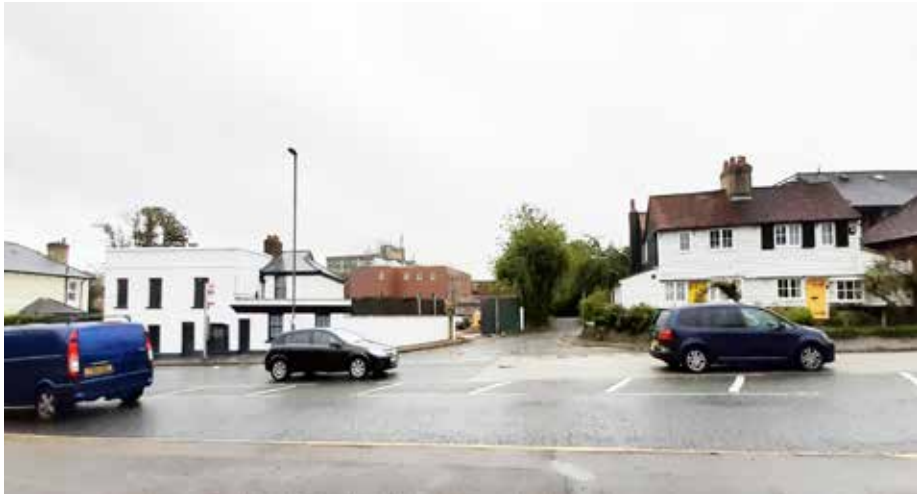
Plate 33 View towards the site with The White Horse and 67-69 Dorking Road in the foreground
