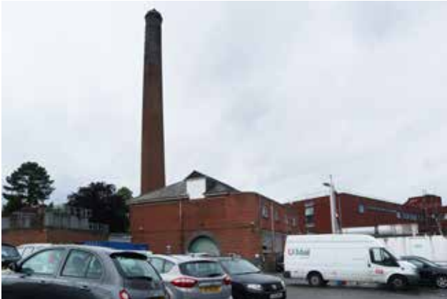
Plate 17 1930s building within the study site
