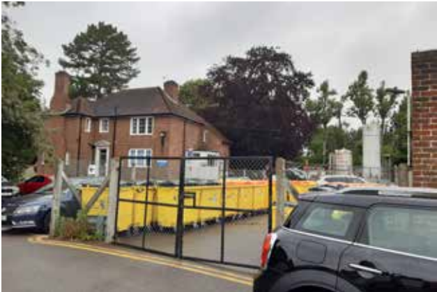
Plate 15 Building in the north western half of the study site used for research purposes
