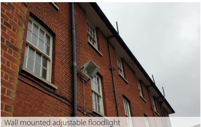
Wall mounted luminaire with downward lighting emission
