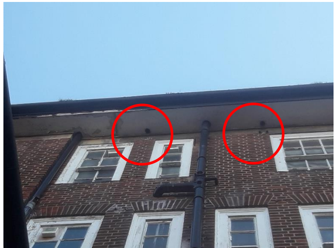
Photograph 6 Rowan House: PRF – Hole in soffit box
