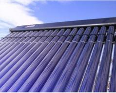
Solar water heating systems use heat from the sun to heat domestic hot water. The system requires solar panels on the roof, ideally south facing, linked to hot water storage cylinders. For solar water panels to be effective the development should have a high hot water demand.
