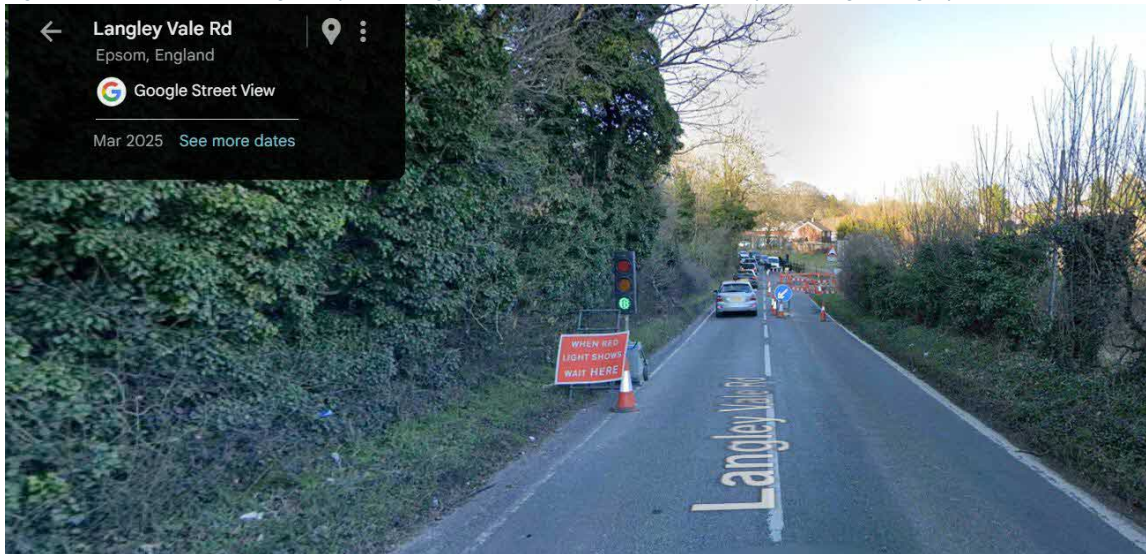
Figure 6-3: Extract from Google Maps showing roadworks in situ in March 2025 (Ref: Google Images)
