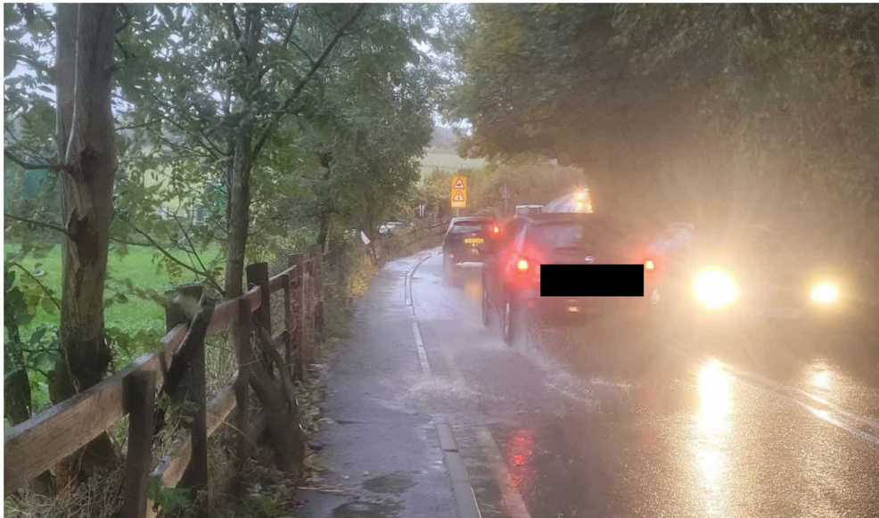
Figure 6-1: Surface water Build-up at the Proposed Site Access (20 th October 2025)
