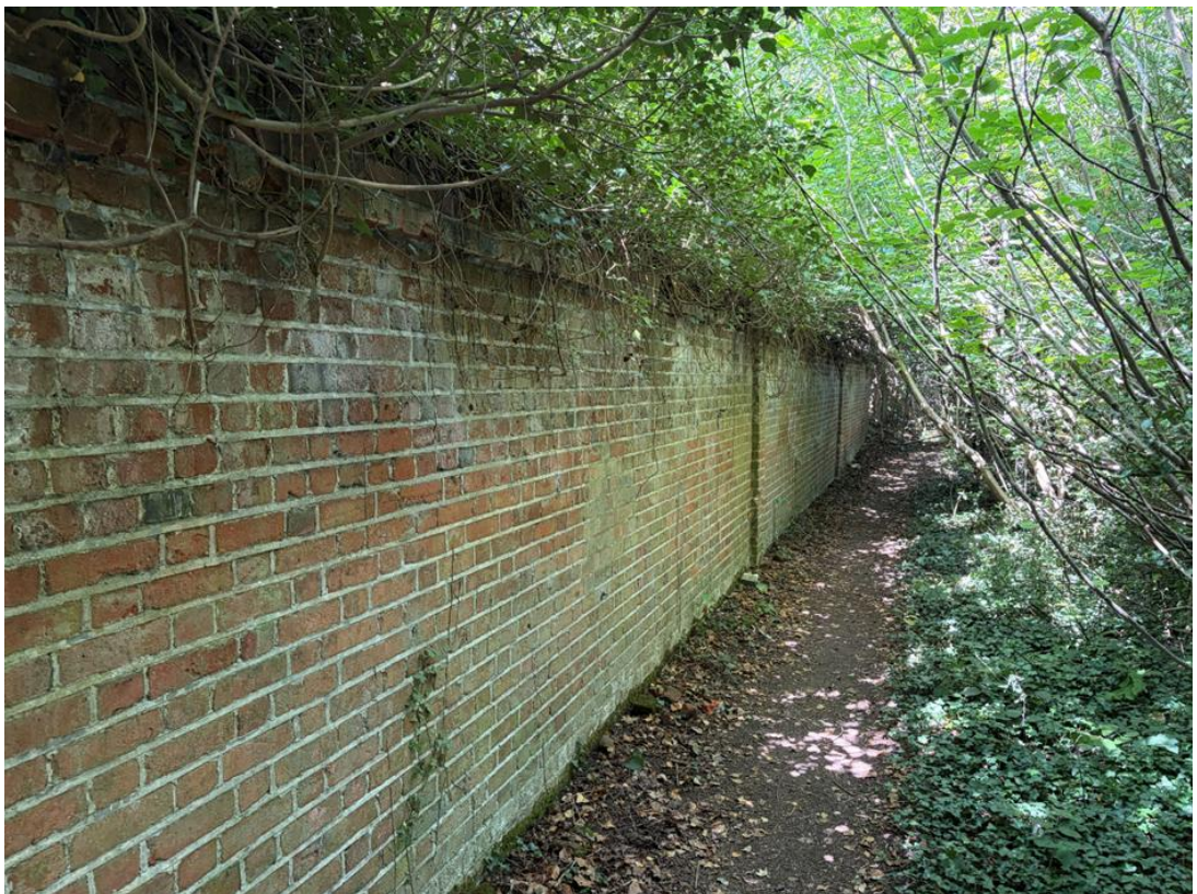
Figures 8 and 9: The South-West Section of the Wall is substantially more intact than the West Section. This is particularly the case at its eastern extent (Figure 9) where the Wall has seen only localised repairs. The western parts have been largely lost, although standalone sections do survive (Figure 8).
