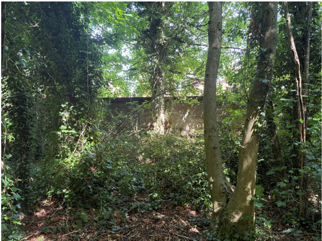
Figures 10 and 11: The North Section of the Wall includes sections that have been rebuilt (Figure 10) and more historic sections that have seen less alteration (Figure 11).
