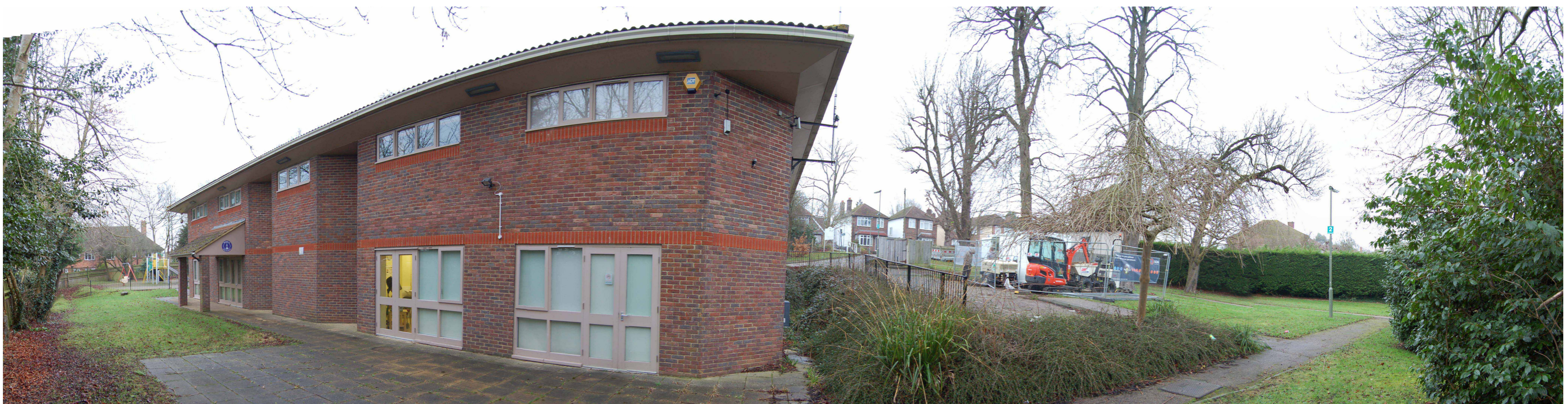
VIEW FROM SOUTH EAST CORNER
