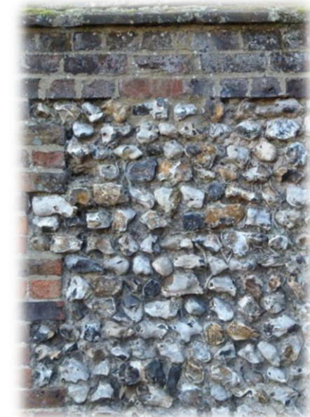
Right: a historic wall in the Church Street Conservation Area illustrating the use of brick and flint.
