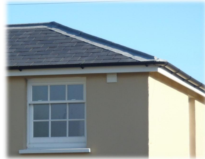
An example showing the use of slate roofing materials and external render in the Pike's Hill Conservation Area.
