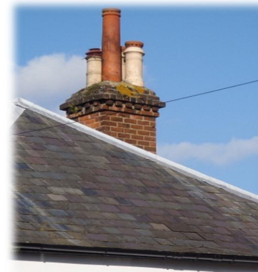
Left: an example of a slate roof found in the Church Street Conservation Area, immediately adjoining the Development Brief site area.
