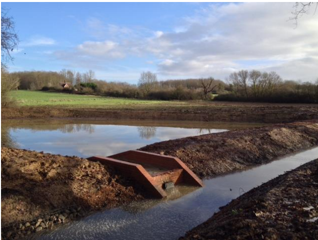
New balancing pond in Horton Country Park LNR just after construction January 2016 and November 2016
