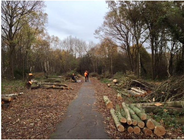
Work taking place to create woodland edge habitat along Pepys Way winter 2016
